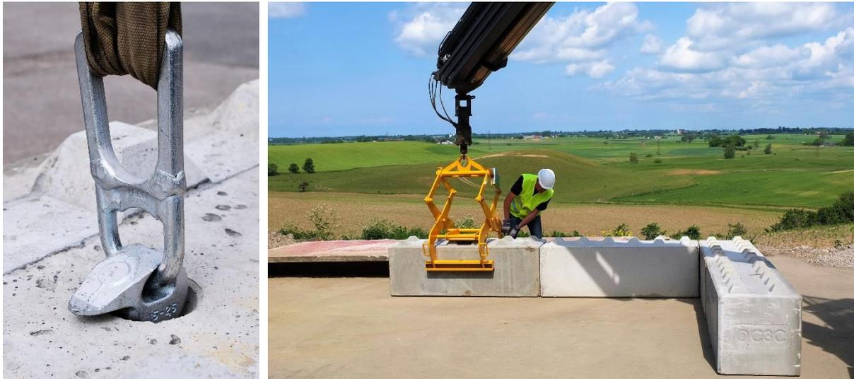
Figure 6.4a-b. Block handling with the help of a universal head lifting link and mechanical lifting device with clamp.
