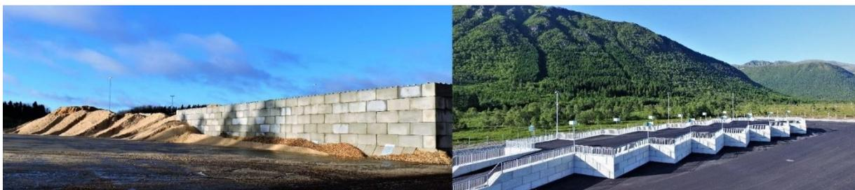
Concrete surfaces are constructed with staining, matrix casting and specific surface treatment for project-specific requirements, in which case the products are manufactured on a project-specific basis to meet the needs of specific projects.
